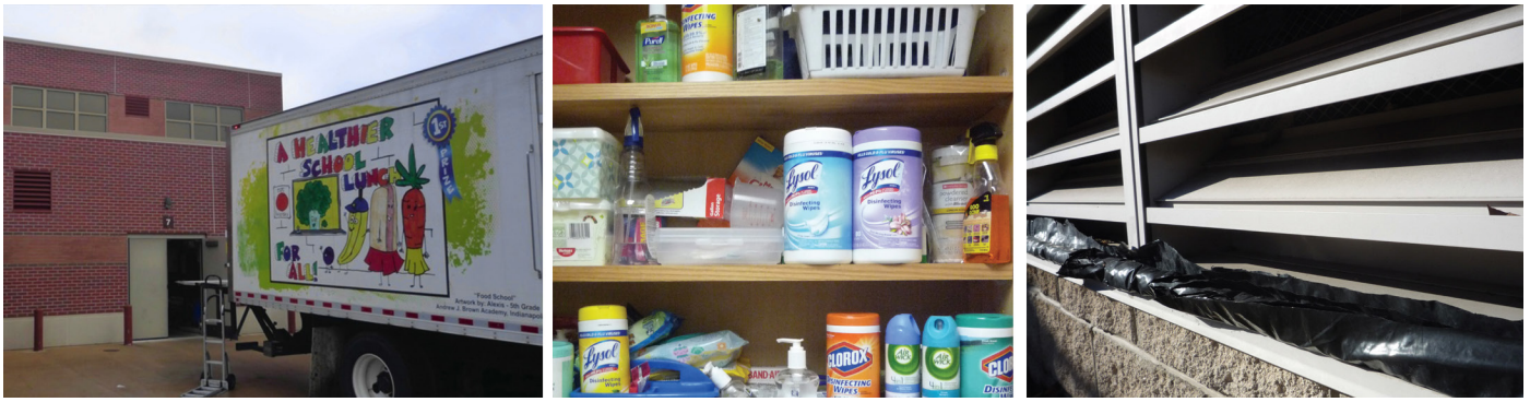
Figure 1: Field Observations (left to right): Delivery truck in a “no-idling” zone adjacent to classroom OA intake vents visible on second floor. Classroom chemicals are a significant concern exacerbated by teachers’ autonomy in operating individual classrooms. Energy saving imperatives often deflect operational logics, example of plastic sheeting applied over OA intake during winter months to reduce energy demand loads. (images courtesy of authors)
