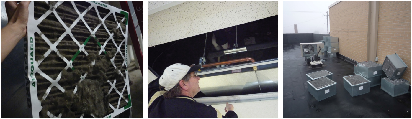
Figure 2: Filter replacement was a consistent concern across school types. In some instances, cost or lack of knowledge regarding replacement protocols was a contributing factor, however ease of access and in some instances access perceived to be dangerous in overhead or rooftop locations was a mitigating factor. (images courtesy of authors)
